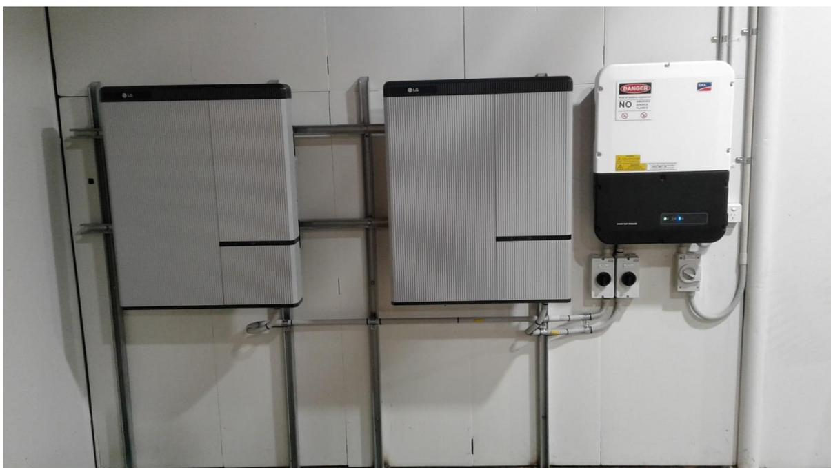
The above photo shows two ten kilowatt LG batteries together with the inverter. The “Unistrut frame was constructed by Lyal and Drew Mitchell it supports the batteries which each weigh around a 100kgs. The installation was carried out Wednesday April 1<sup>st</sup> and by Thursday both batteries were fully charged.
